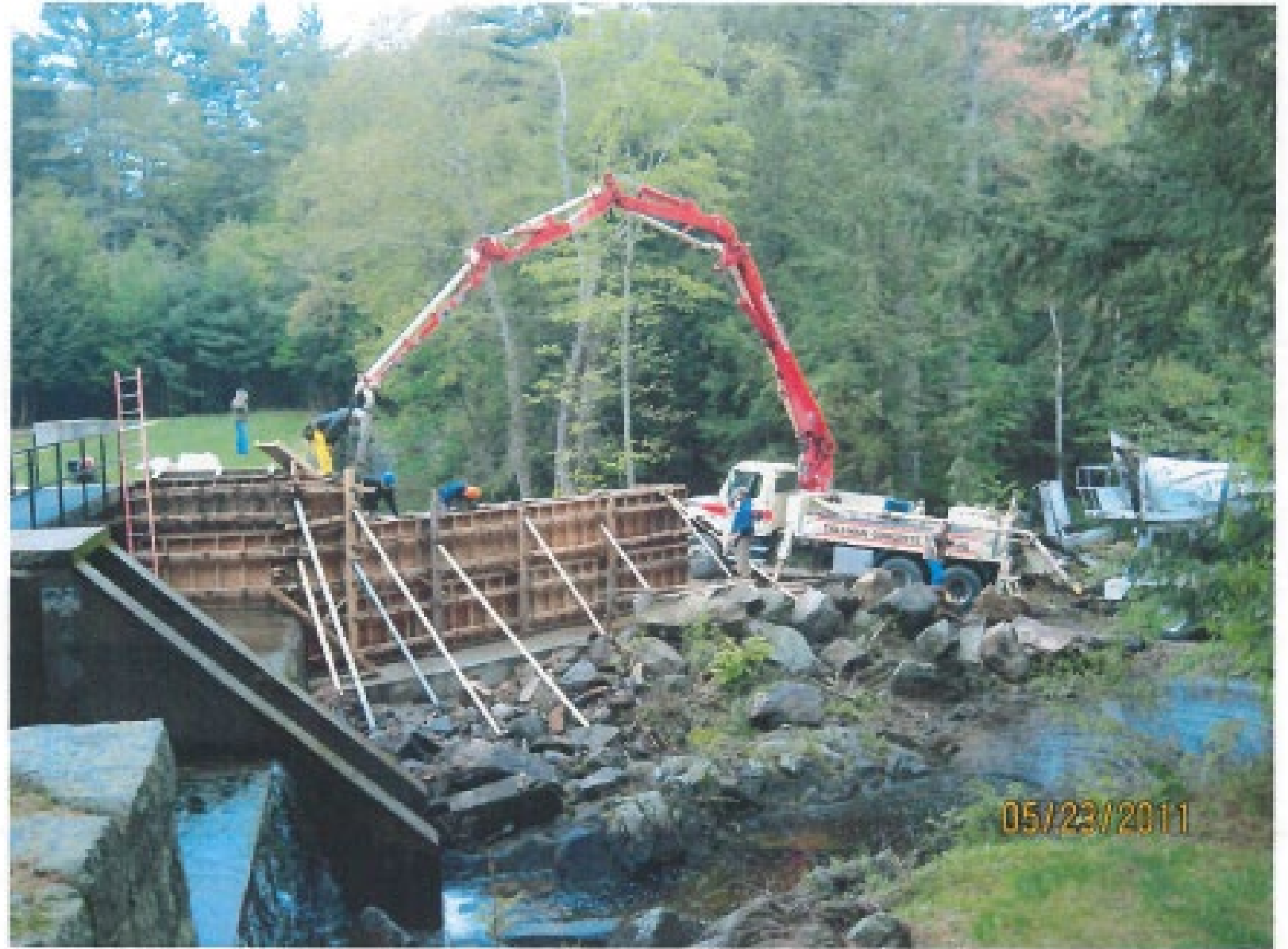
Photograph 5 – Concrete pumper truck used for wall pour.
