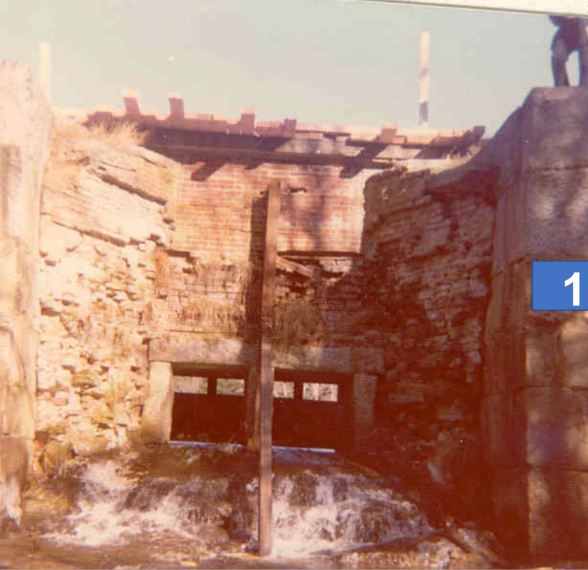
Original stoplog spillway section built in 1956 (1974 photo)
