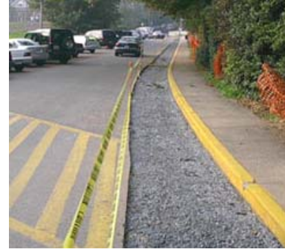
A stone-filled infiltration trench constructed to intercept runoff from the adjacent road.
